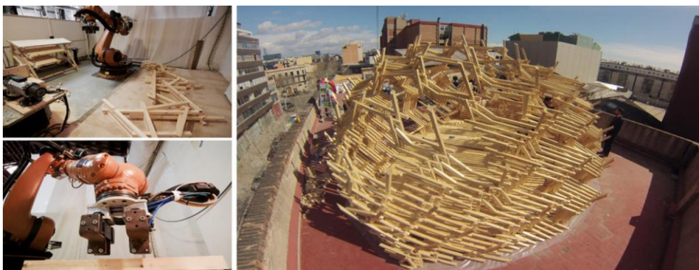
Figure 2. An adaptive robotic fabrication process makes possible a necessary scaling-up and handling of complex interrelations between the pattern shapes and the behaviour of novel materials. In contrast to repetitive manufacturing processes where automation relies on the execution of predetermined and fully defined steps, sensing technology enables a workflow that synthesizes material computation and robotic fabrication in real-time. In this process, the shape of the tailored workpiece is repetitively scanned.
