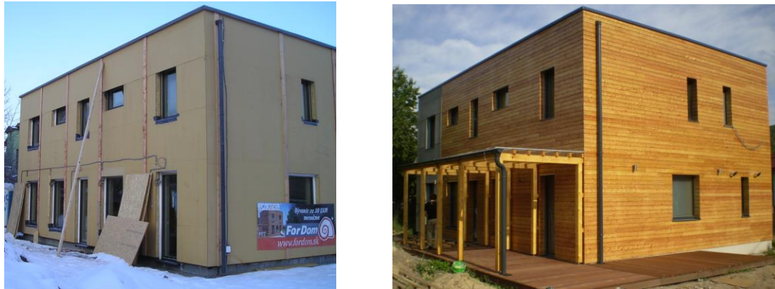
Figure 4. The case study house (left-during construction, right – finished house)
