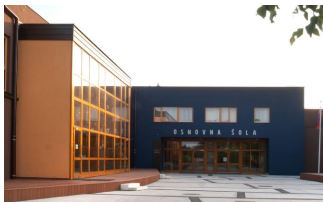
Figure 1. Reused wooden beams as a new evacuation staircase of the Primary School Brezovica (Osnovna šola Brezovica). Author of the project: Slavko Gabrovšek (foto Slavko Gabrovšek).
